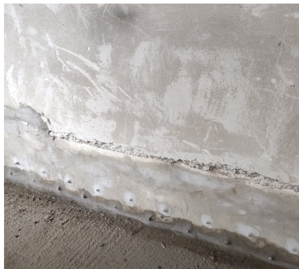
Slika 6 Prikaz ojačanja unutarnjih zidova FRM mrežom Figure 6 Illustration of the reinforcement of internal walls with FRM mesh
