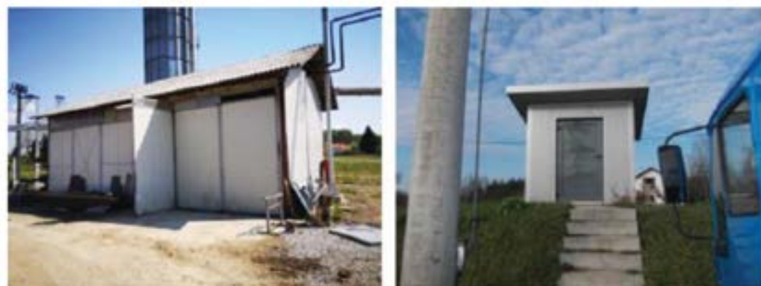
Slika 4 Spremište i podzemni spremnik sa požarnom stanicom Figure 4 Storage and underground tank with fire station
